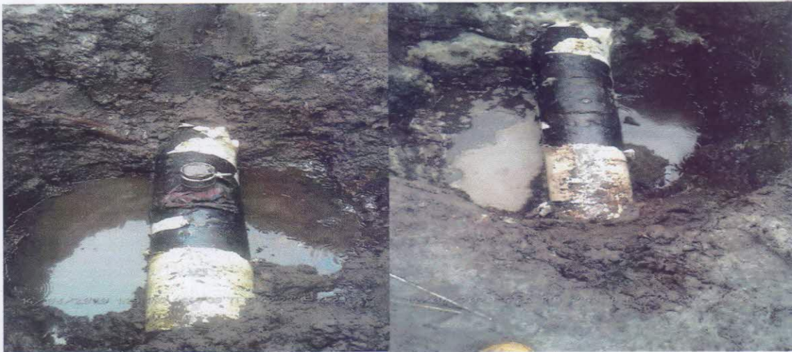
Pictures 1&2 showing installed valve at spill point and repaired point.
